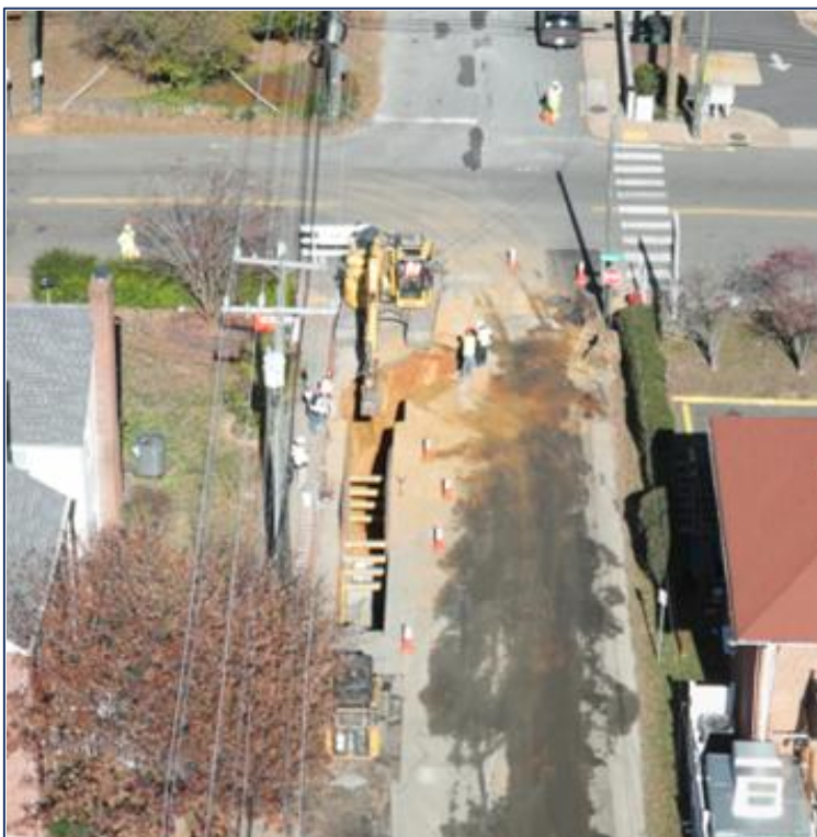
Waterline installation on Lewis Street
